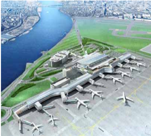
Source: created by the Company based on material from the Tokyo International Air Terminal Corporation
