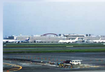
Terminal 1 goes into operation.
