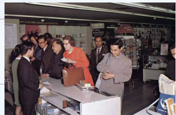
Japan's first duty-free shop. With the 1964 Tokyo Olympics approaching, the terminal is expanded and given a new look.
