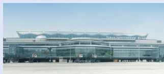
Terminal 3 (PFI Project) Opens
