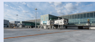
Terminal 2 North Satellite
