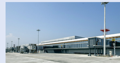
Terminal 1 North Satellite
