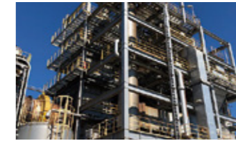
Waste incineration facility
