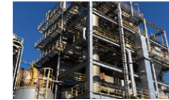
Waste incineration facility
