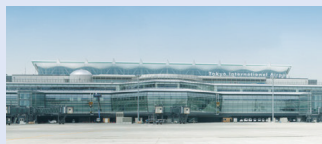
Terminal 3 (PFI Project) Opens
