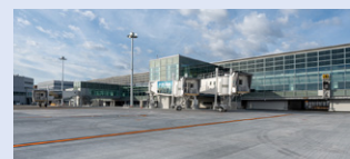
Terminal 2 North Satellite
