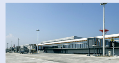
Terminal 1 North Satellite
