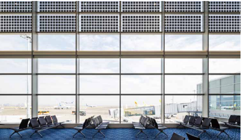
The installation (interior)
