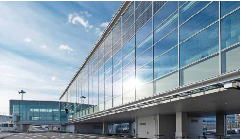
The installation (exterior)
