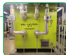
Geothermal heat pump chiller
