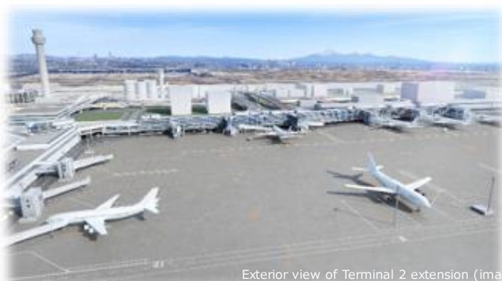
Exterior view of Terminal 2 extension (image)
